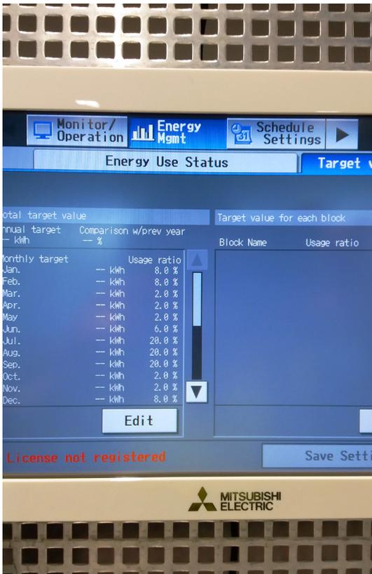
**An advanced MelcoRemote control system has been installed to monitor the energy use of both the VRF and Hybrid VRF systems, along with the Ecodan heating units, lighting and extract fans within the building.**
