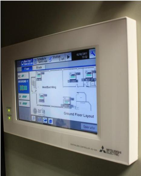
AG150 touch screen centralised controllers were added to maximise energy efficiency, decrease energy usage and minimise running costs.
